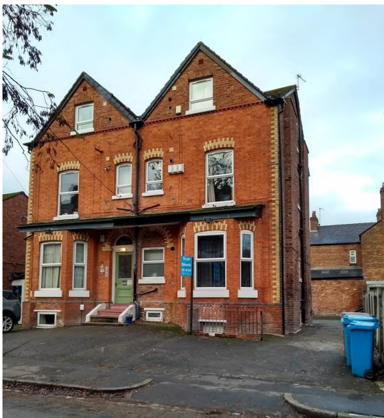
Semi's converted to flats on Northen Grove – loss of gardens and boundary walls
