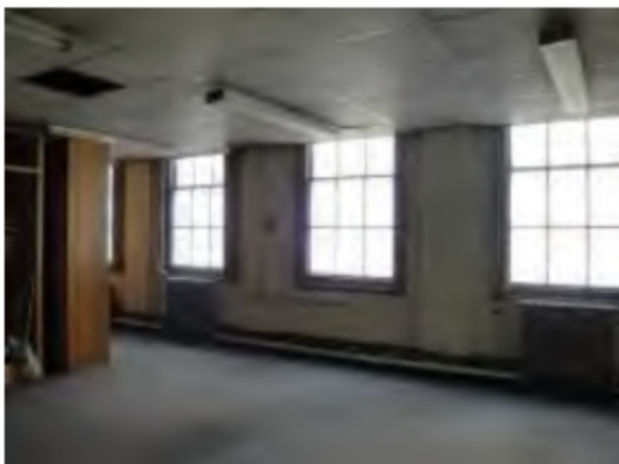
Subdivision of the former office spaces at first floor level
