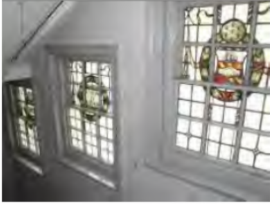
Example of the leaded glass windows to the stairwell.
